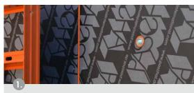
Errection of the formwork (Outer formwork with clamping unit, inner formwork with quide bushing)
