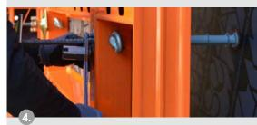
Lock the guide bushing and screw the guide bushing with the assembly tool
