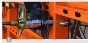
Feed the tie rod, tube and guide bushing through the inner formwork, turn the tie rod into clamping unit
